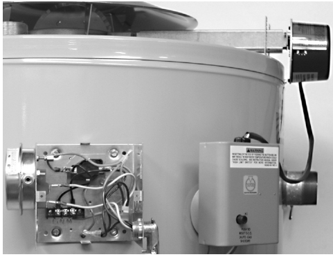
(1) Mount the CK-41P Control Kit near the appliance.
