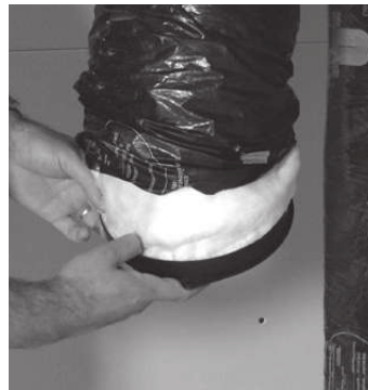
Figure 7.2 Insert insulation inside the collar.
