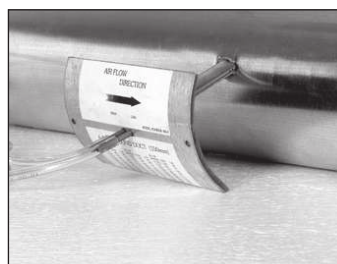
Inserting Air flow grid in duct
