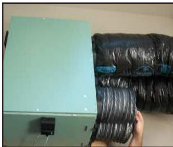
Figure 7.4 Slide collar on the unit.
