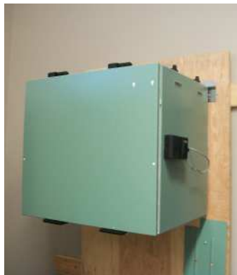
Figure 6.2 Hang HRV/ERV to wall mounting bracket.
