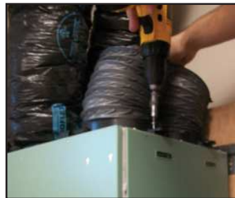
Figure 7.5 Fix and secure the collars to the HRV/ERV with the #10 x 1 1/4" screws, supplied in kit.
