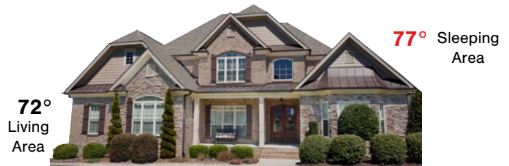
In two-story homes, upstairs sleeping area feels too warm during the summer
